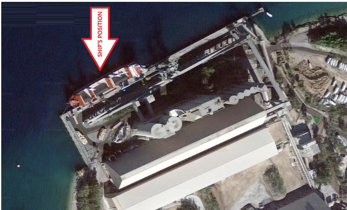
Fig. 3.3/1: Indicative picture of the ship's position at the time of the marine casualty, moored alongside at the port facility of Titan Group at Drepanon , Achaia, Greece (Source: Google Maps)
